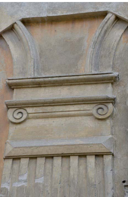
A detail of stucco decoration of the school building facade (House of Study)
