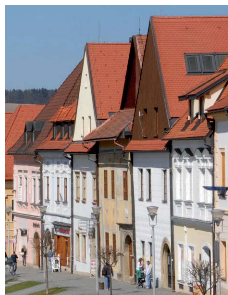
Restored burgher houses in the southwestern side of the Town Hall Square
